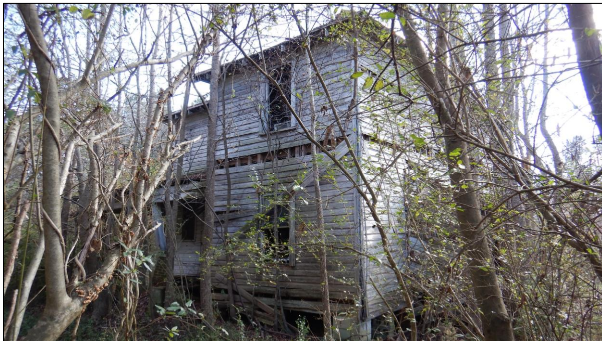
Figure 7. NP0537, dwelling facing southeast.
