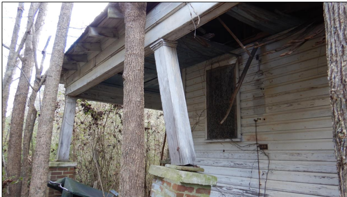
Figure 9. NP0537, dwelling porch column details, view southeast.
