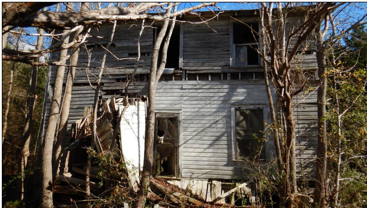
Figure 11. NP0537, dwelling west elevation with collapsed entryway and porch, view east.
