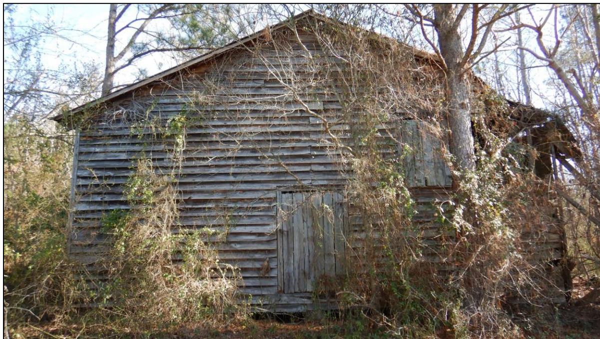
Figure 15. NP0537, barn facing east.
