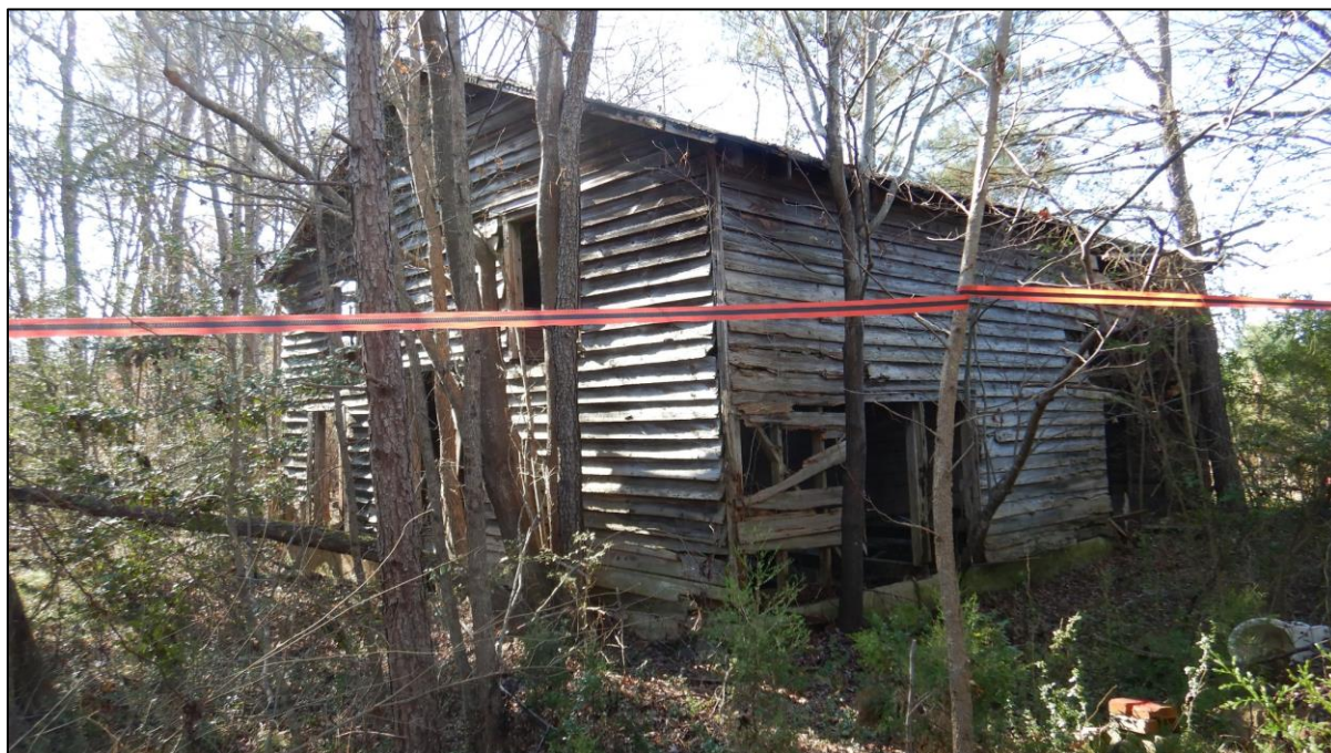
Figure 14. NP0537, barn facing southwest.
