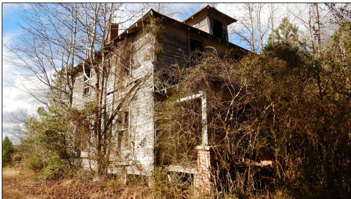
Figure 4. NP0537, dwelling facing northwest.
