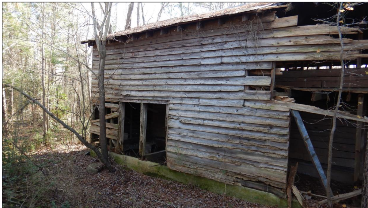
Figure 13. NP0537, barn facing south.
